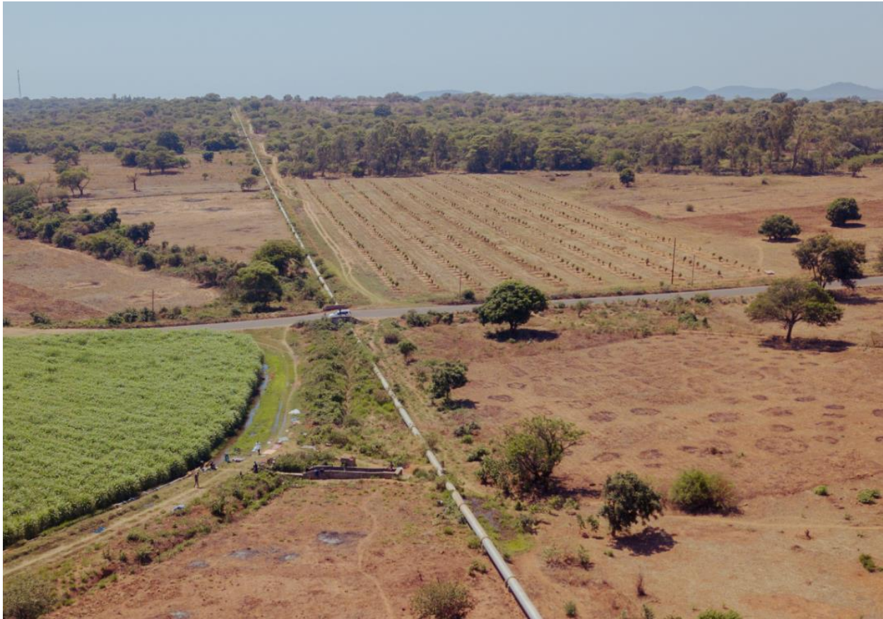
Figure 23. Drone imagery, main pipeline to KASCOL (03-12-2021)
