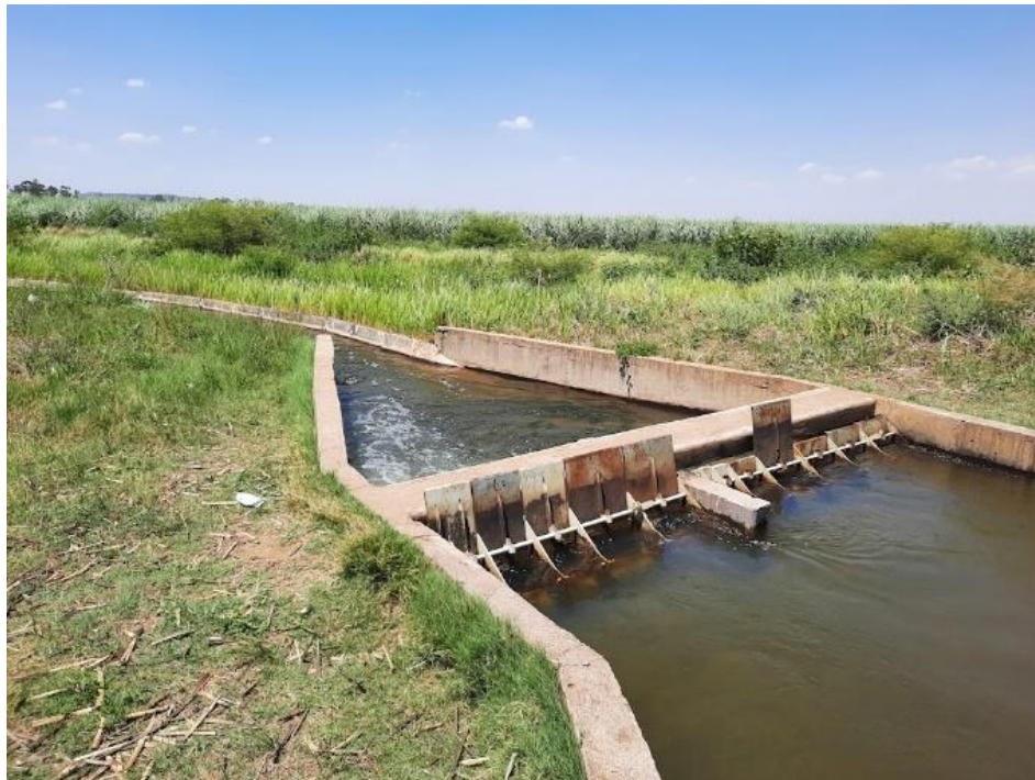
Figure 13. Calibrated undershot gates in open canal furrow irrigation system at Kaleya farm (03-12-2021)
