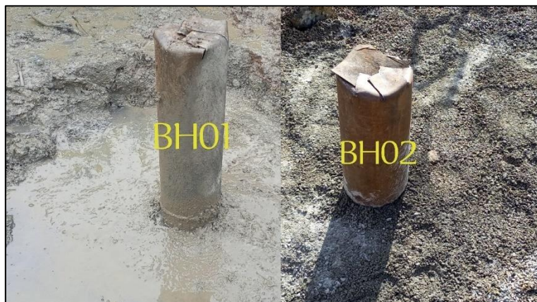
Figure 7. The two Boreholes sealed after completion of works
